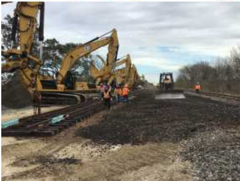
WT Byler railroad crews assist Union Pacific Railroad with the installation of #20 Turnouts on the mainline at the Crosby-Dayton Railroad Project.
