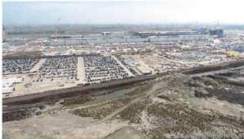
Progress on Samsung's chipmaking plant in Taylor as of Dec. 2023.
